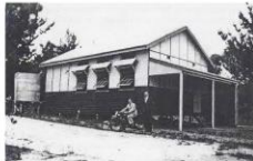
IMAGE 02: CARMARTHEN SCHOOL IN SITU 1940
