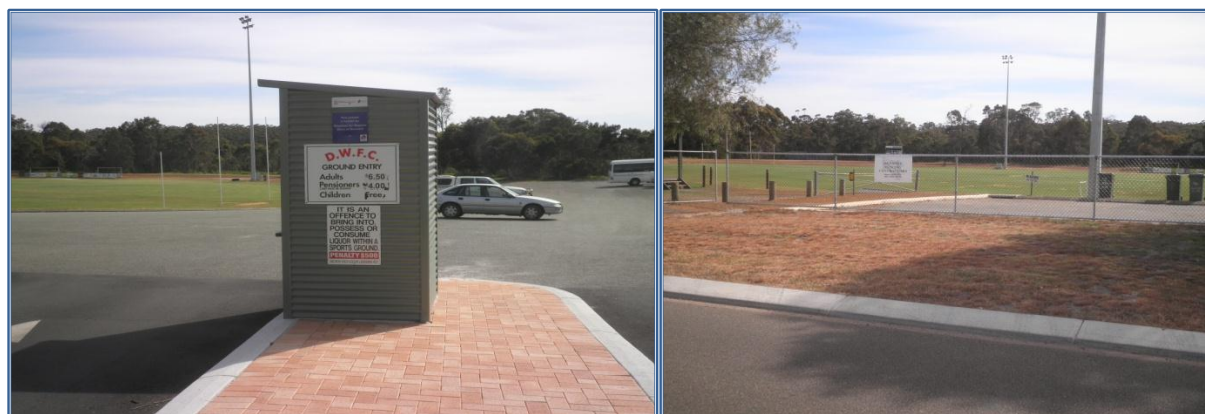
McLean Park facilities from Brazier Street
