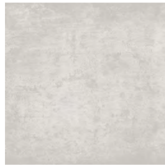
Grey smooth & sand blasted concrete
