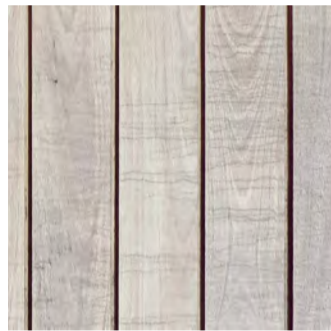
Weathered timber battens & screens
