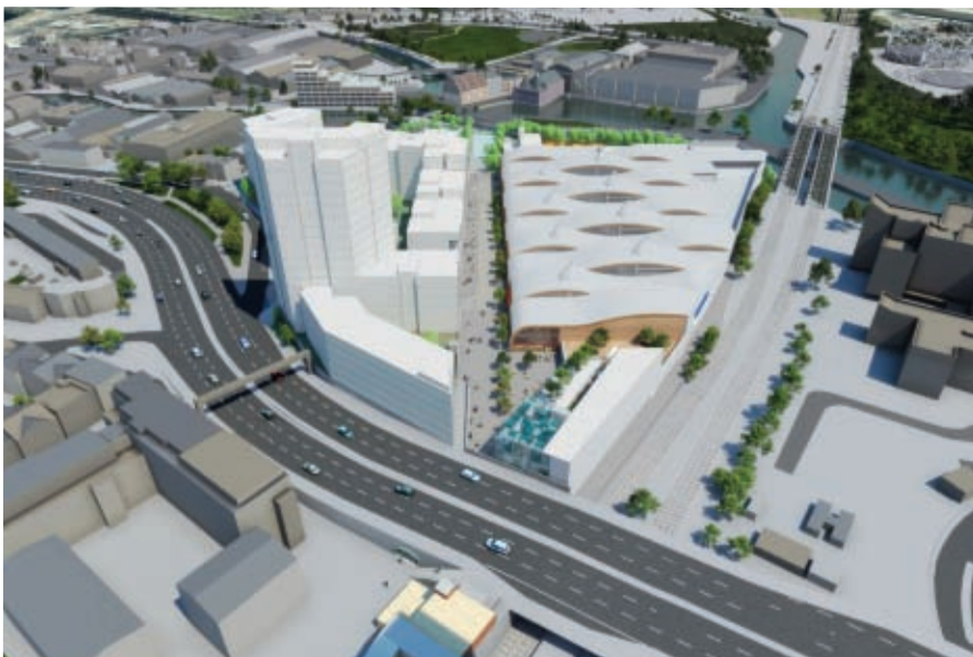
This scheme in Bromley-by-Bow, east London is complex superstore-led regeneration which is driven by the Tesco-led investment opportunity, even though planning and design guidance underpins the scheme. The site layout gives precedence to the supermarket, which enjoys a river frontage. The residential tower will be sited where noise, air quality and outlook are at their worst, beside the northern approach to the A12 Blackwall Tunnel
