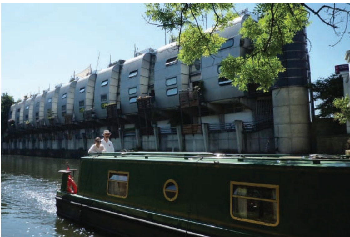
Grimshaw's Grand Union Walk housing scheme for Sainsbury's in Camden was completed in 1988 and it is still a desirable place to live. Residential units take the form of individual houses, capitalising on the canalside setting. The south facing wall to the rear needed to be blank to exclude lorry noise, so their living space at first floor level is top lit. A double-height dining area opens out onto a balcony
