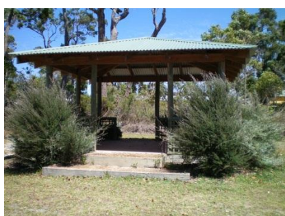
Figure 5 - Gazebo at the Denmark Cemetery along pathway (Pinnaroo)
